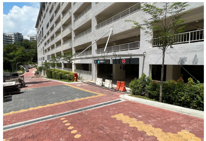
Tower F (Along the slope)
