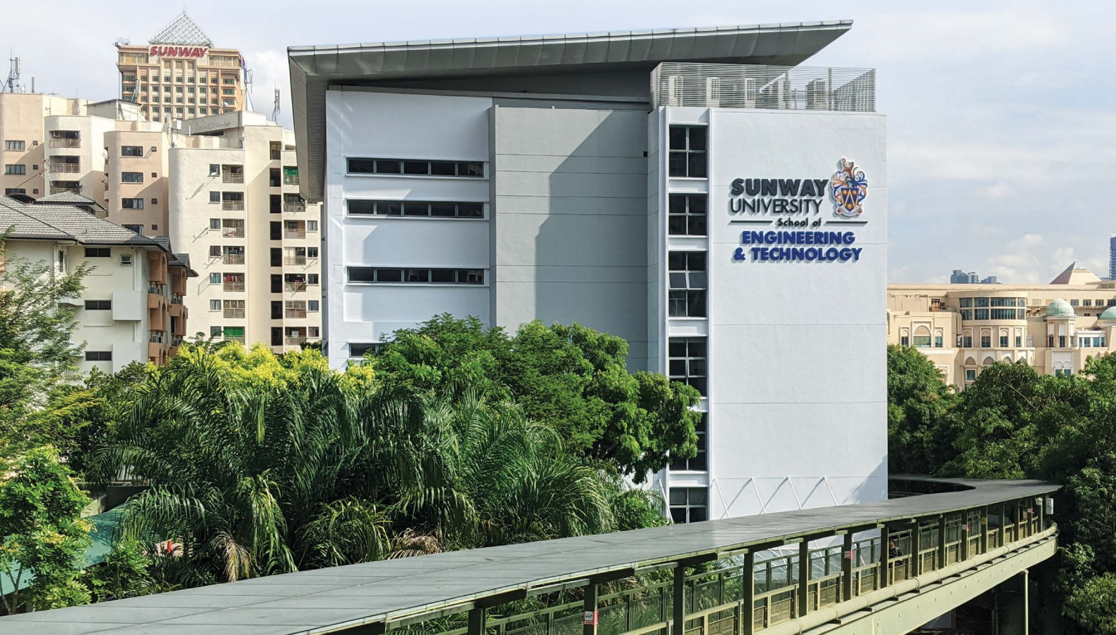
School of Engineering & Technology (SET) Labs building
