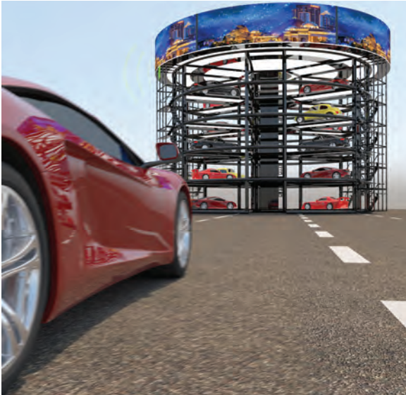
| An empty parking space will be transferred to the car park entrance as soon as the car nears the car park
